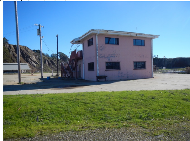
Photo 8. View facing east at the Operations Building located at IR Site 4 (Drum Lot 1) (February 1, 2016; Map 13).
