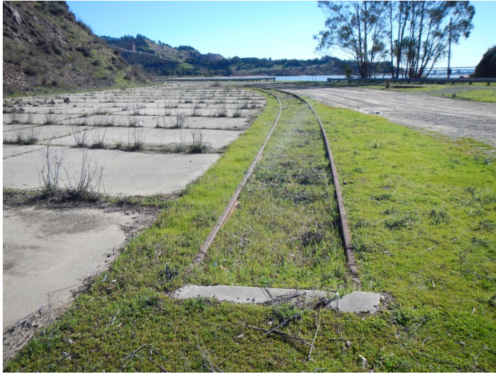
Photo 29. View facing south at the former railroad corridor in the eastern portion of IR Site 4 (Drum Lot 1) (February 1, 2016; Map 13).
