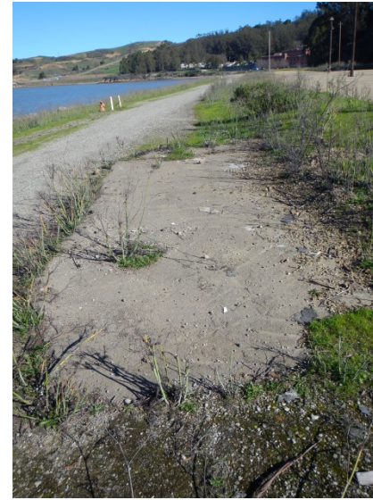
Photo 6. View facing northeast at the northwest portion of IR Site 4 (Drum Lot 1). What appeared to be asbestos roofing shingles were observed in this area (February 1, 2016; Map 13).
