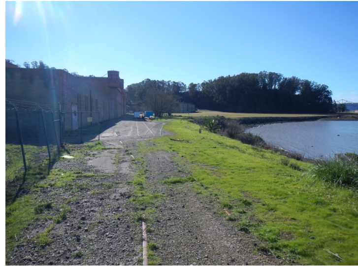
Photo 2. View facing south at the former railroad corridor. Building No. Warehouse is located in the left hand portion of the photograph (February 1, 2016; Map 16).
