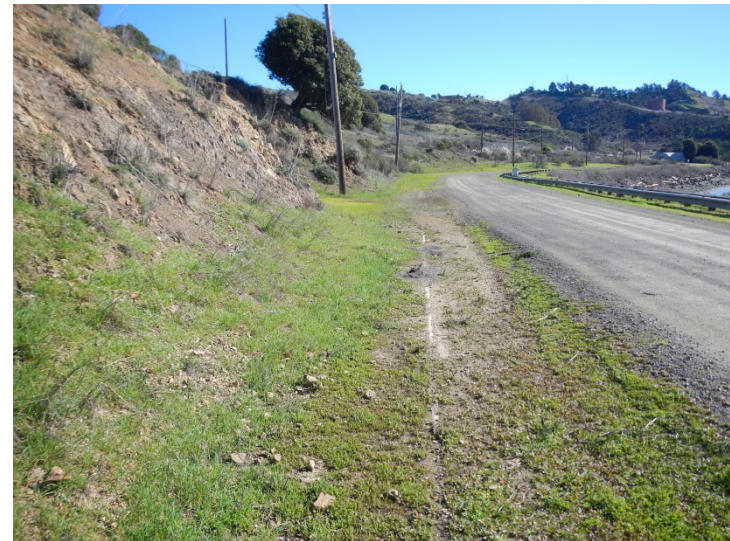
Photo 24. View facing east at former railroad corridor (February 1, 2016; Map 12).
