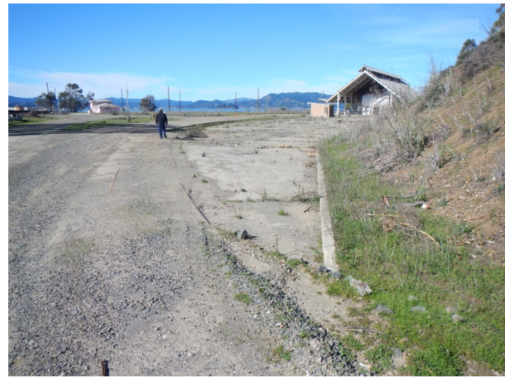
Photo 28. View facing north at Building 89 Lube Oil Store (February 1, 2016; Map 13).
